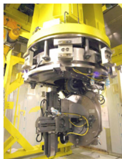
F9 - Sodium Reactor Decommissioning
