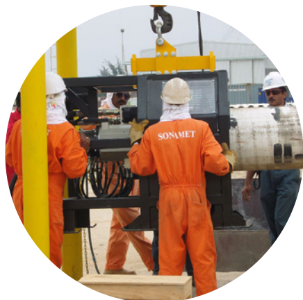
Concentric clamping jaws for a perfect alignment of the tubes.
