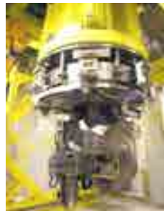
F9 - Sodium Reactor Decommissioning
